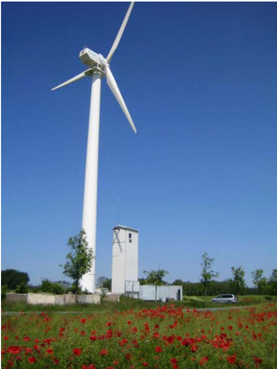
Fig. 3.: MVC-plant with a vertical tube evaporator-condensor-unit.
